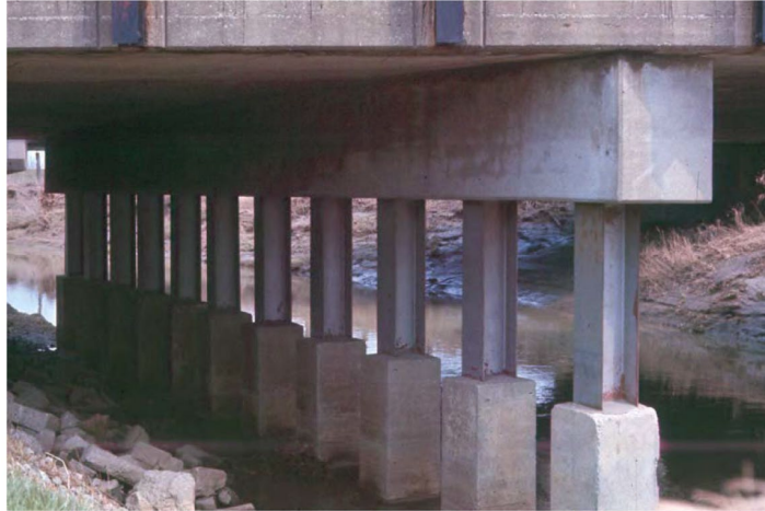
Figure 1.5 Concrete encasement retrofitting method (ODOT 2008).
