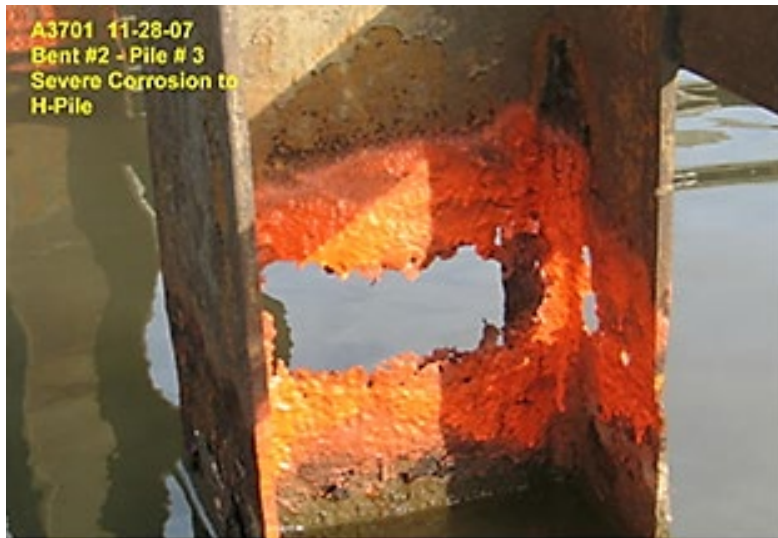
Figure 1.2 Corroded steel column.
