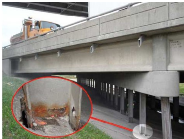
Figure 1.1 Corrosion of H-piles in I-70/I-270 interchange in St. Louis.
