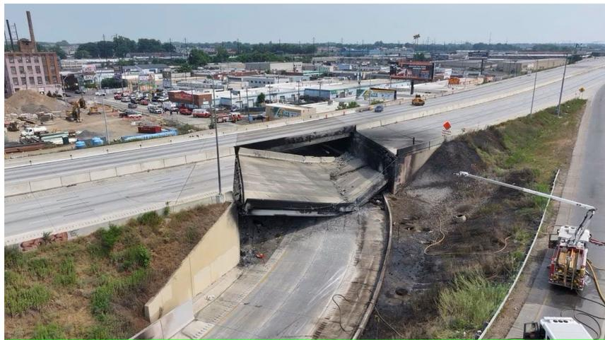
Figure 2.24 Collapse of a part of I-95 highway after a multi-hazard incident, Philadelphia, Pennsylvania (Tebor and Sottile 2023)
