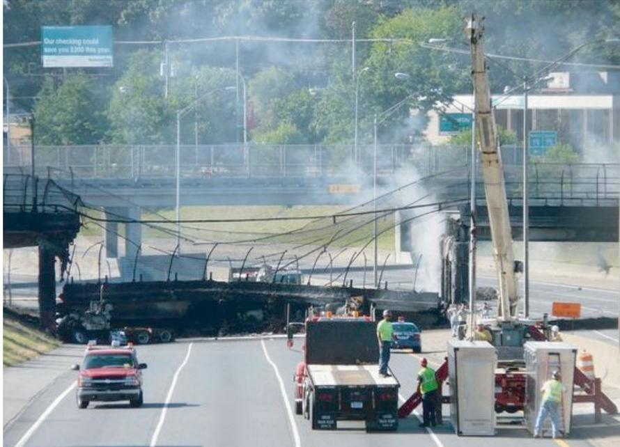
Figure 2.19 Hazel Park bridge overpass collapse as a result of fire, Detroit, MI (Guthrie, Goodwill, and Hicks 2009)
