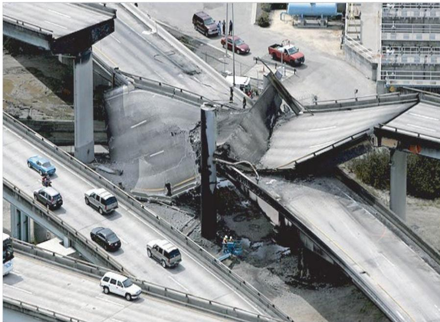
Figure 2.18 Highway bridge collapse as a result of fire, Oakland, CA (Bulwa and Fimrite 2007)
