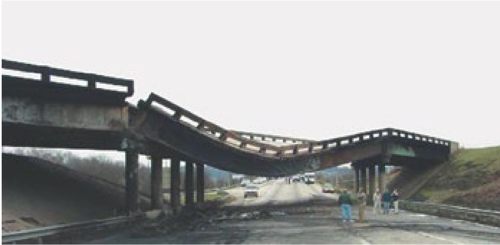
Figure 2.25 Damage in I-65 bridge overpass caused by multi-hazards, in Birmingham, Alabama, 2002 (Cardone, 2023)
