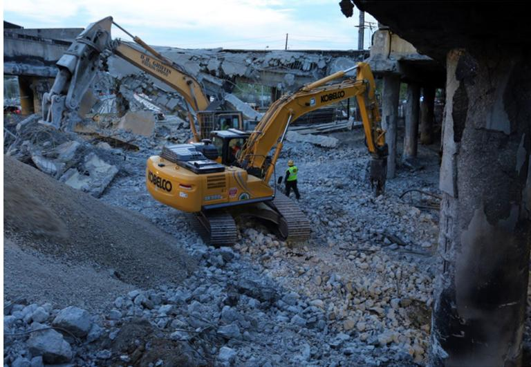
Figure 2.21 Post fire damage to I-85 bridge, Atlanta, GA (Venkatesh Kodur and Naser 2021)
