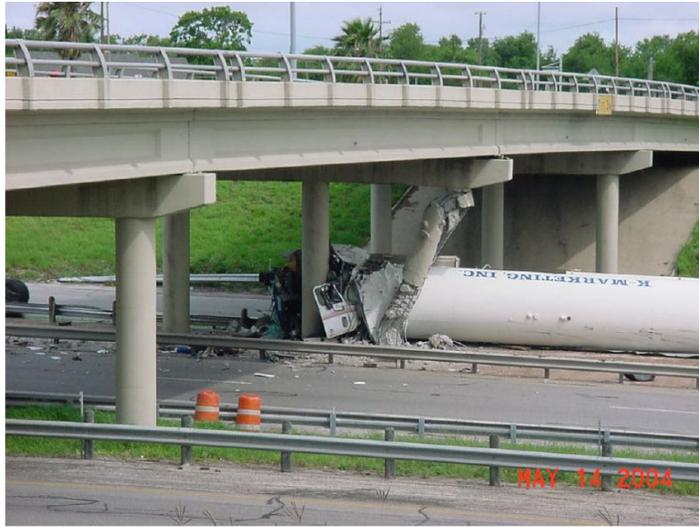
Figure 2.7 Tanker truck pier collision, I-37, Corpus Christi, TX (Buth et al. 2010)
