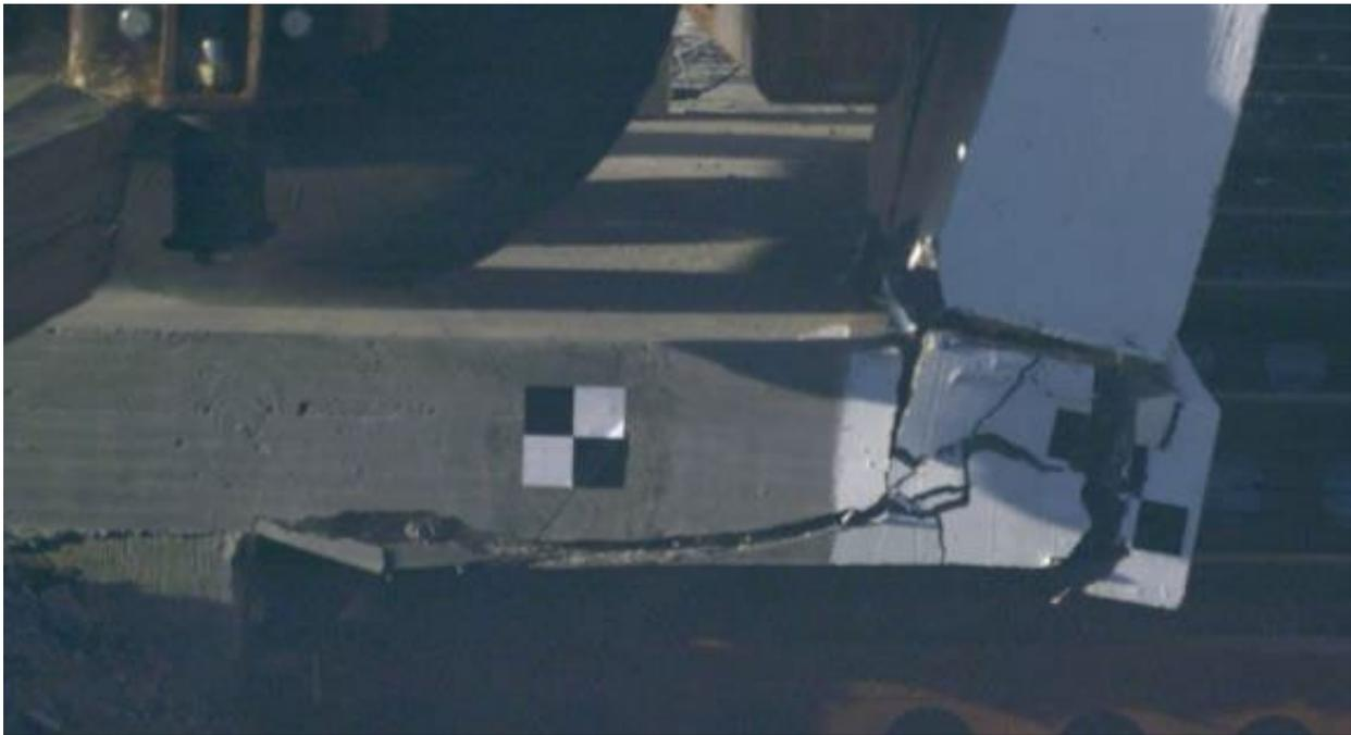
Figure 6.10 Damage in bridge deck supporting concrete parapet railing
